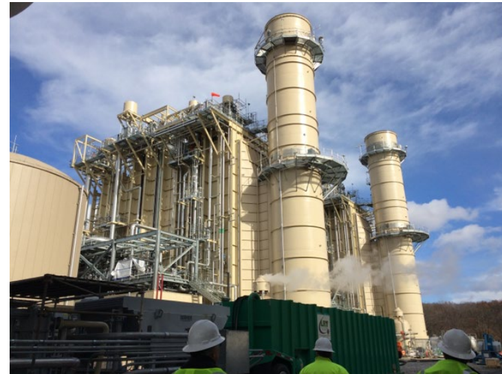
Electric Generating Facilities
