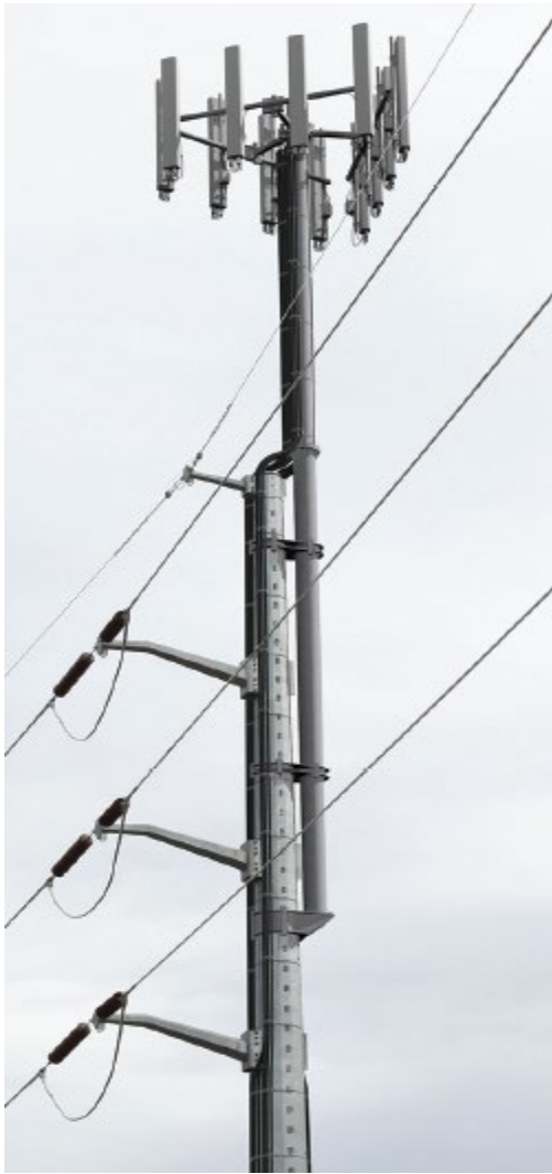
Transmission Line structure mounted antenna arrays
