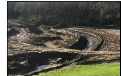
Construction in progress. Natural tributary on the left. Relocated ditch on the right. Natural tributary to be filled in after construction.
