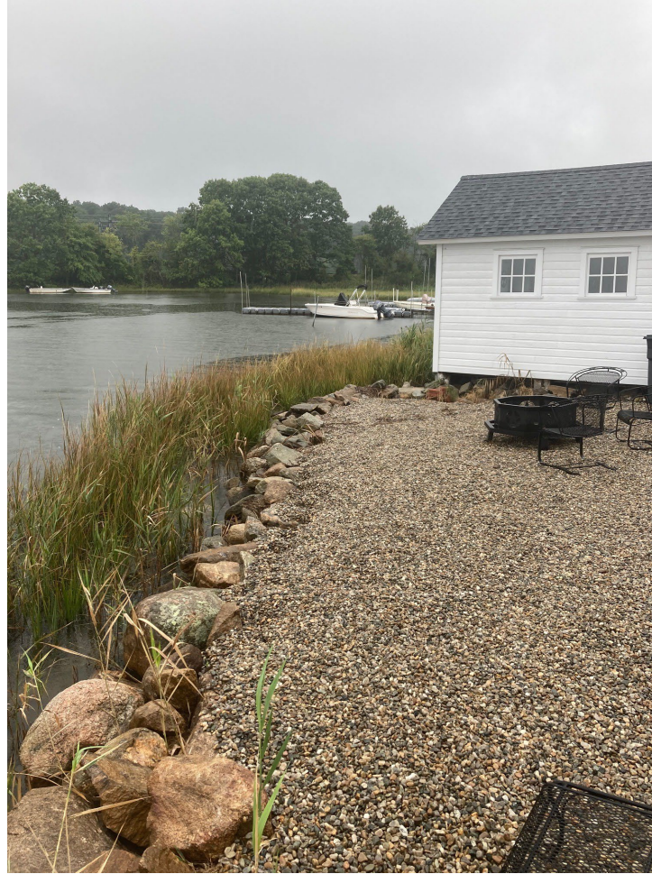
New gravel fill and rip rap
