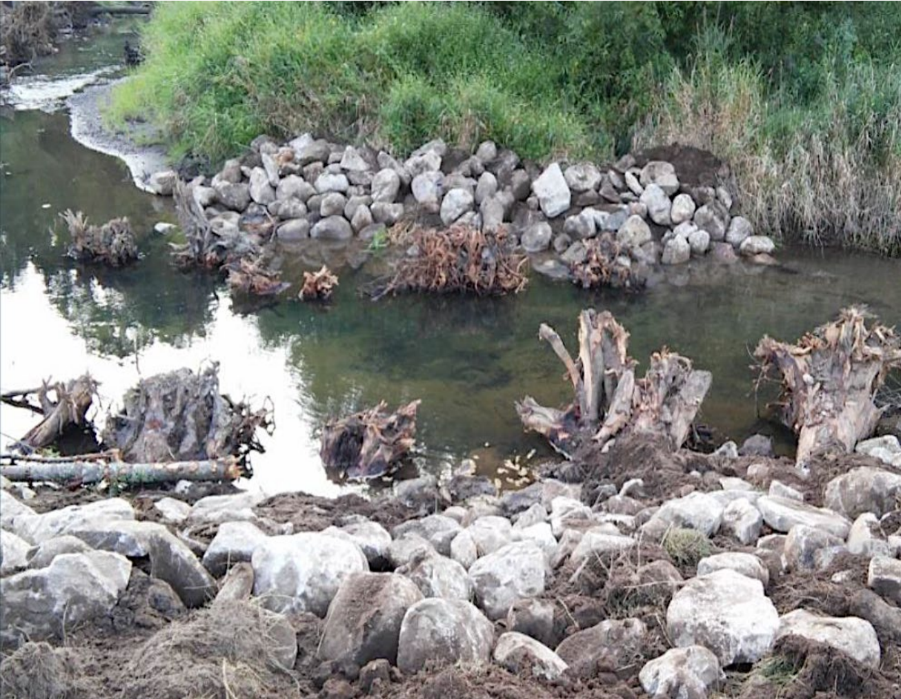
Thermal pool treatment on the Salmon Kill, Salisbury, CT
