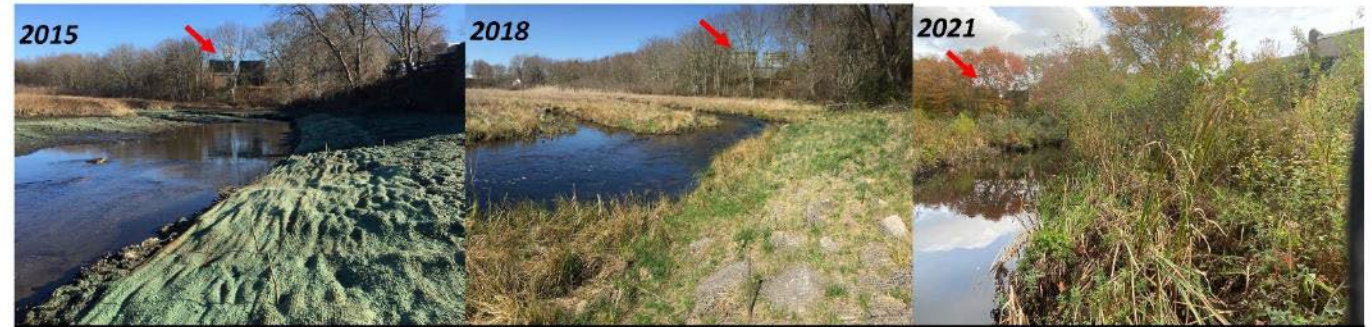
EXAMPLE: Channel Bank Reconstruction at Hyde Pond Dam Removal, Mystic, CT:
